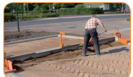
Screeding of 5.5 meter accurately between kerb and gutter.
