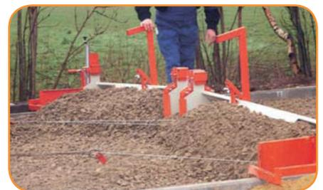
Screeding of coarse gravel mixture with central elevation (Crown)
