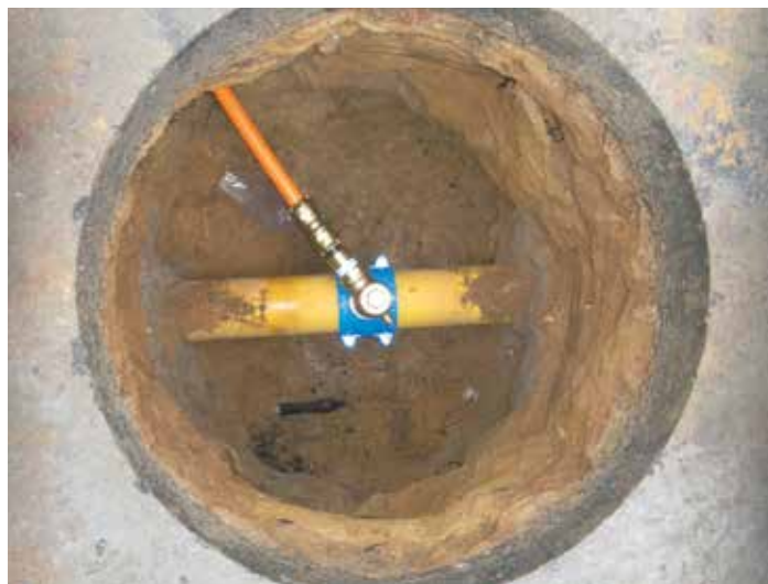
Completed connection
