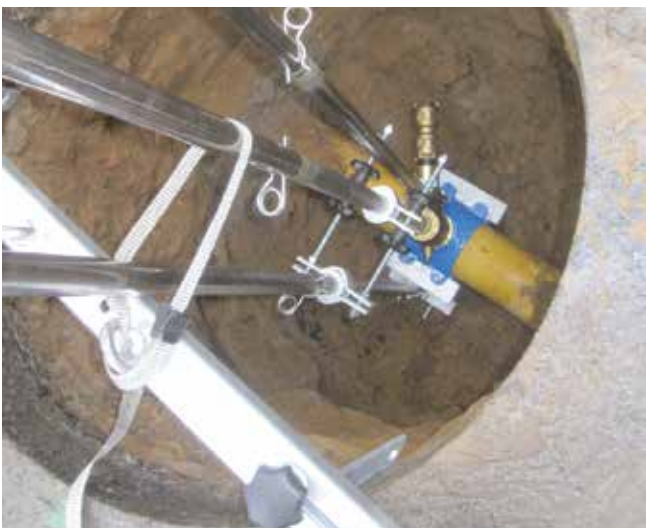
Assembly of connection fittings.
