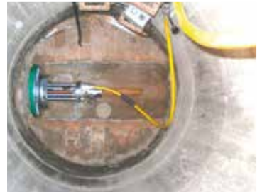
BURSTFIX 200 inside the manhole
